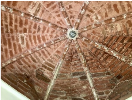
Brick vaulted ceiling of the private Chapel
